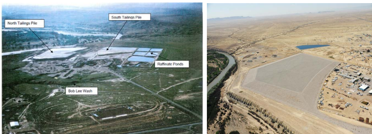
Figure 37 Aerial View of the Shiprock UMTRA Site in 1965 and after Completions of Disposal Cell in 1986 Disposal Cell
