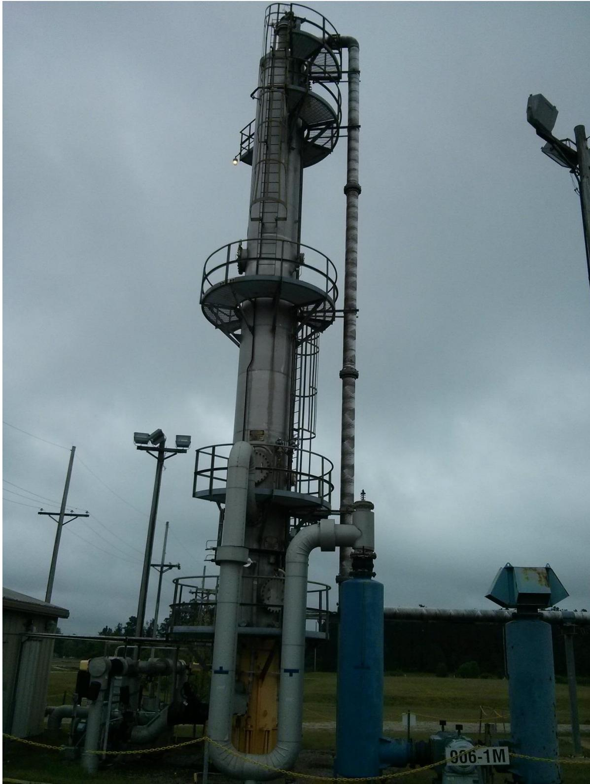
**Figure 1. Photograph of the full-scale M1 air stripper at the M-Area, SRS.**
