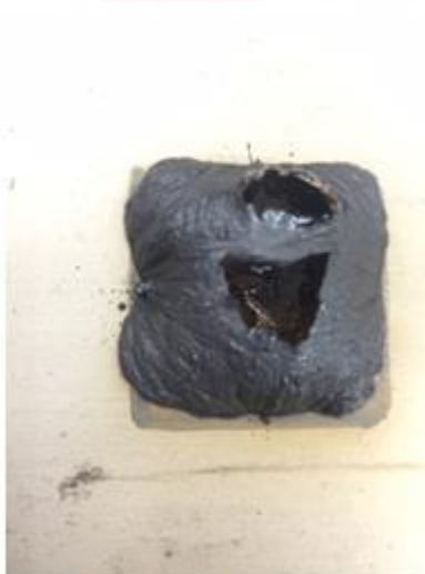
Significant discoloration, continued expansion and "off gassing", mass loss, desiccation, cracking, and brittle composition (700 degrees)
