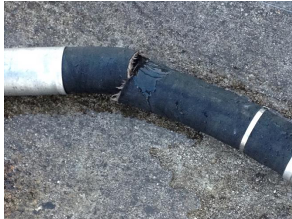
Figure 7. Ruptured hose section.
