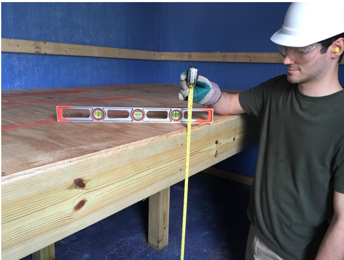
Figure 8. Construction of SRS 235-F Hot Cell Test Bed at FIU ARC.
