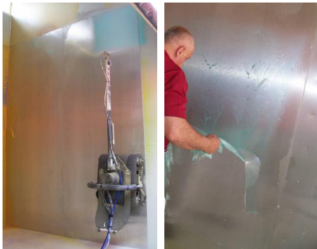
Integrated remote spraying platform - scaling up a vertical wall in building module and applying DeconGel to metal panel. Dry DeconGel peeling from metal panel.
