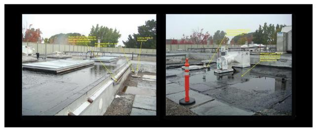
Figure 16. Roof failure at LLNL B251 (Source: LLNL 2013)
