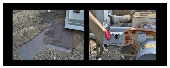
Figure 17. Roof failure at LLNL B292 (Source: LLNL 2013)
