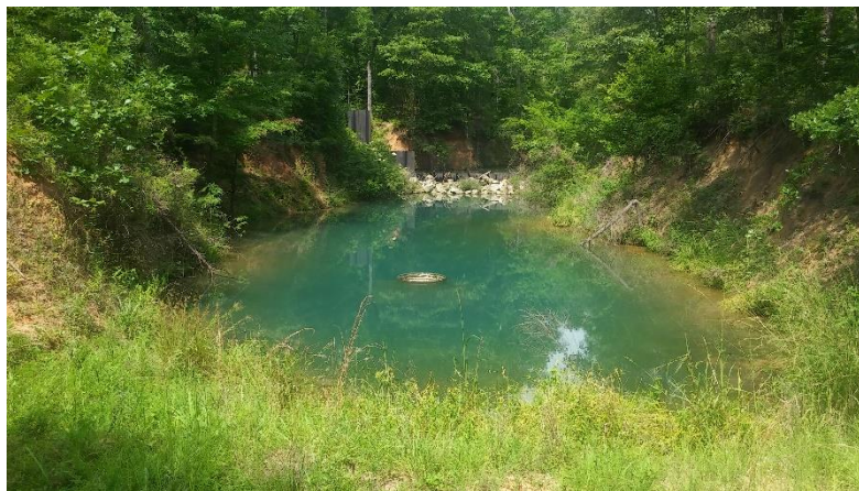
Weir and culvert
