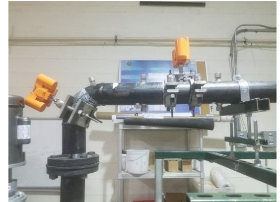
Coupons on the pipe loop
