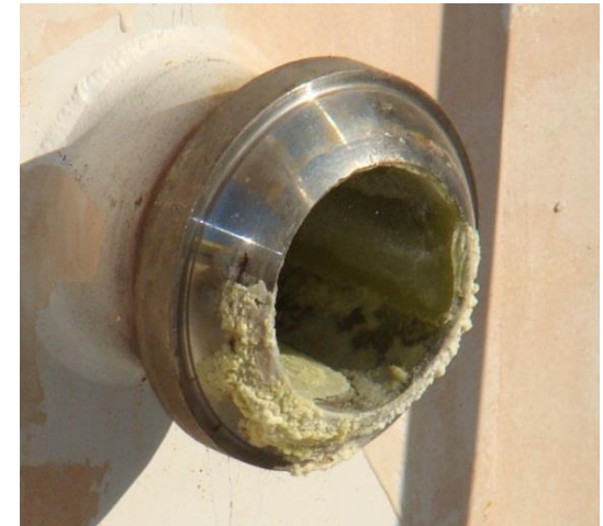
Supernatant Dried on Nozzle 18 in AP Valve Pit.
