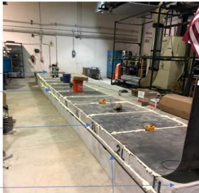
Insulation foam installed at all the cracks
