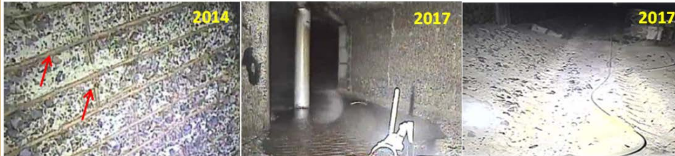
Steel (arrows) and coarse aggregates exposed
