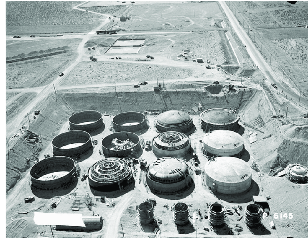
1944 aerial view of the single-shell tanks (SST) under construction at Hanford site C-Farm.
