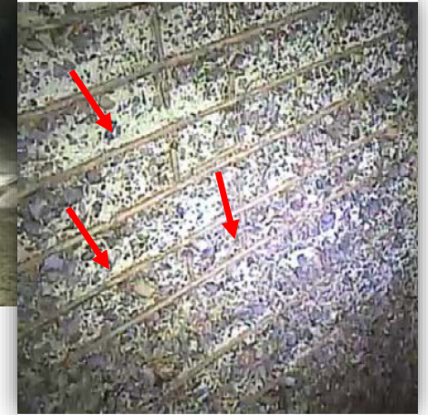
Degraded concrete exposing the steel rebar (red arrows).
