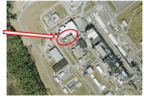
Aerial view of Potential Hot Site at F-Area
