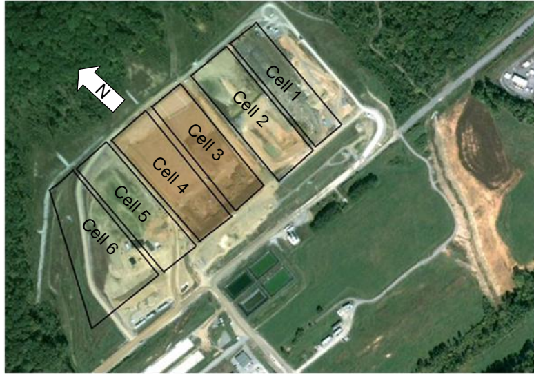
Figure 9. Aerial photo of EMWMF and disposal cells.
