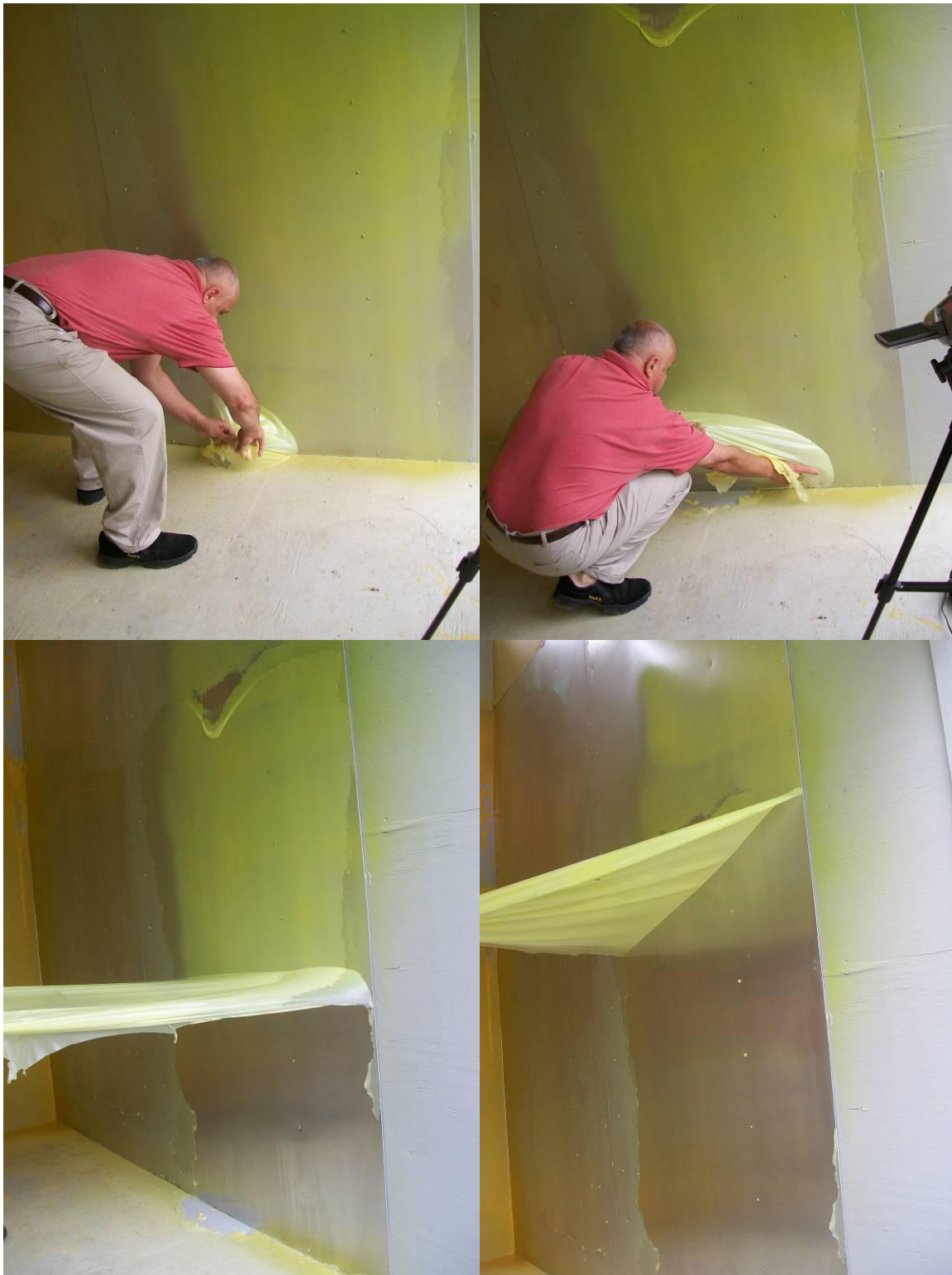
Stripping CC Strip from steel panel (applied during demonstration).
