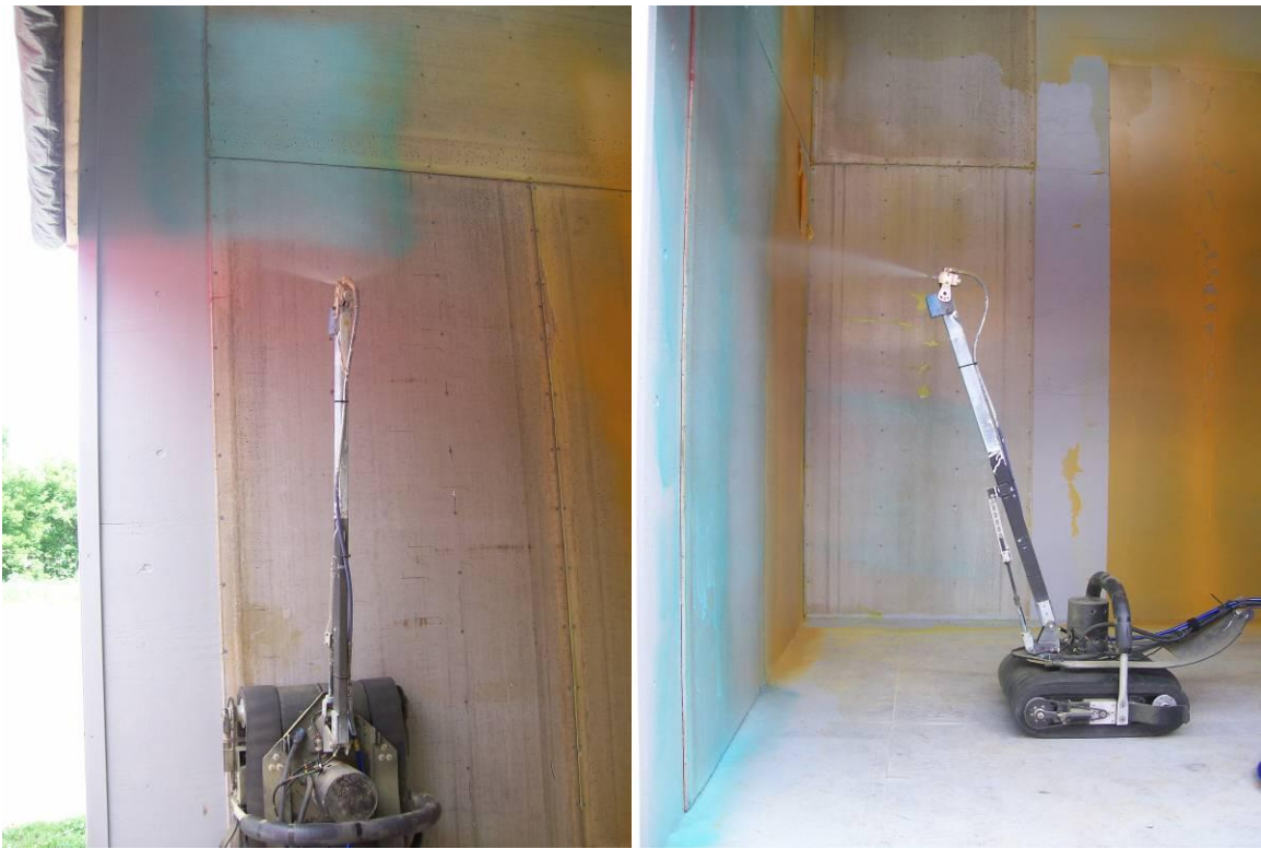
Spraying DeconGel on concrete panel.
