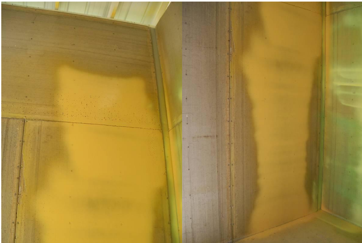
ALARA 1146 sprayed on concrete panel.
