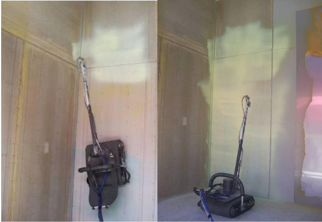
Spraying CC Strip on concrete panel.
