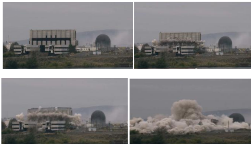
Figure 26. Explosive demolition of Buildings 337 and 337B at the Hanford Site.
