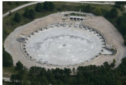
CT aerial at completion
