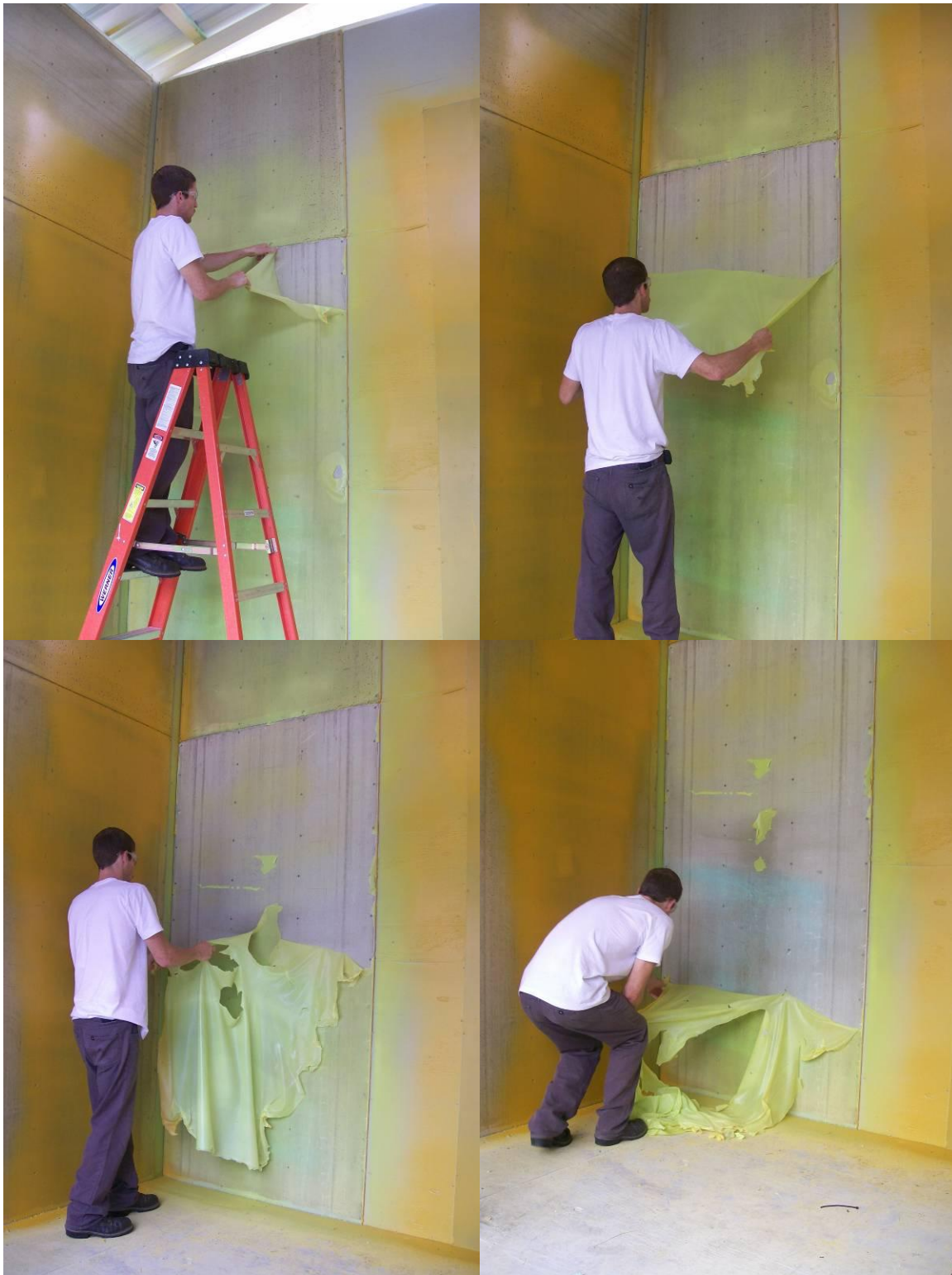
Stripping CC Strip from concrete panel (applied during demonstration).
