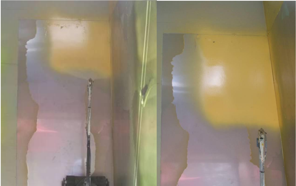
Spraying ALARA 1146 on steel panel.
