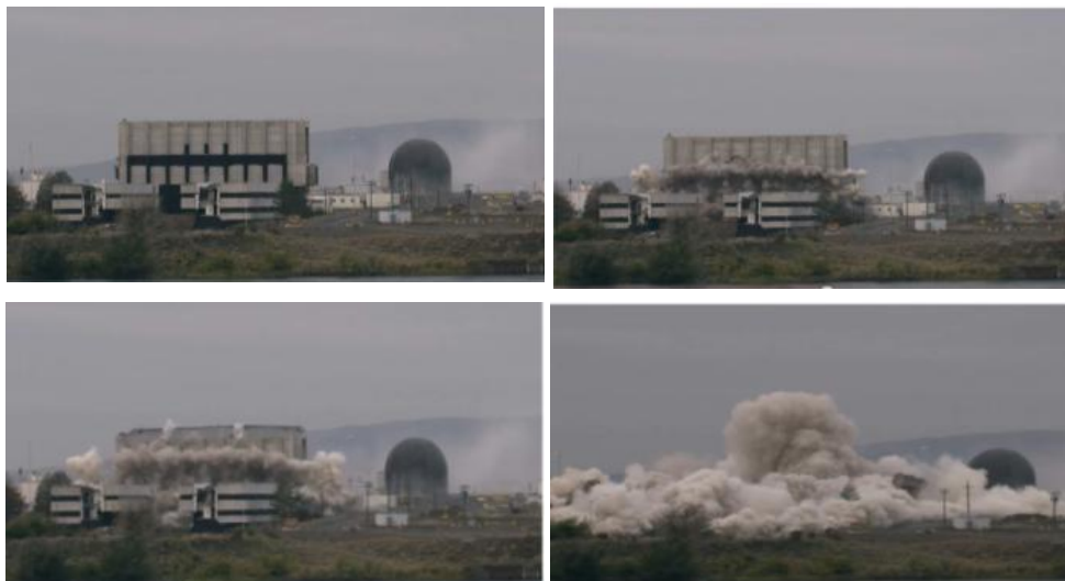
Figure 66. demolition of Buildings 337 and 337B at the Hanford Site.
