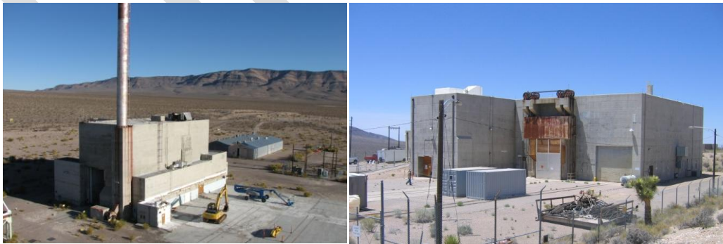
R-MAD Facility (left) and Pluto Facility (right)
