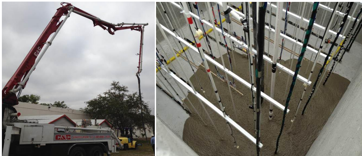
Figure 12. Grout pump and filling the cube with grout.
