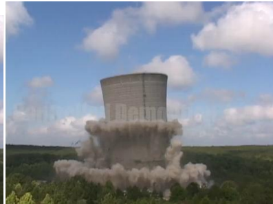
Cooling Tower (during)
