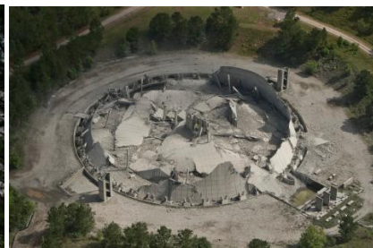
Cooling Tower (aerial, after)
