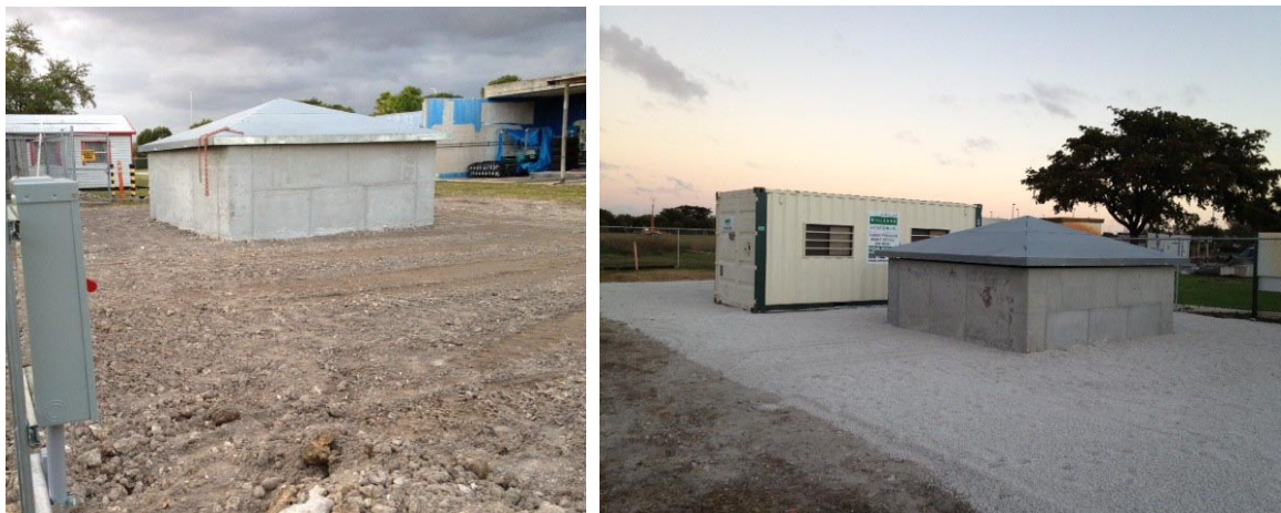
Figure 10. Preparation of the test site.
