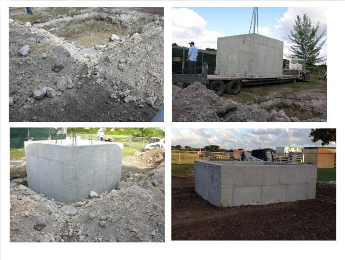
Figure 9. Installation of Cube
