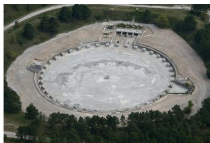
Cooling Tower (aerial, at completion)
