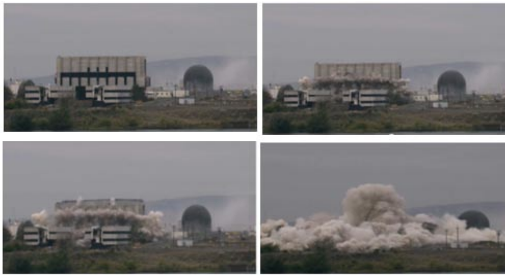
Figure 16. Demolition of Buildings 337 and 337B at the Hanford Site.
