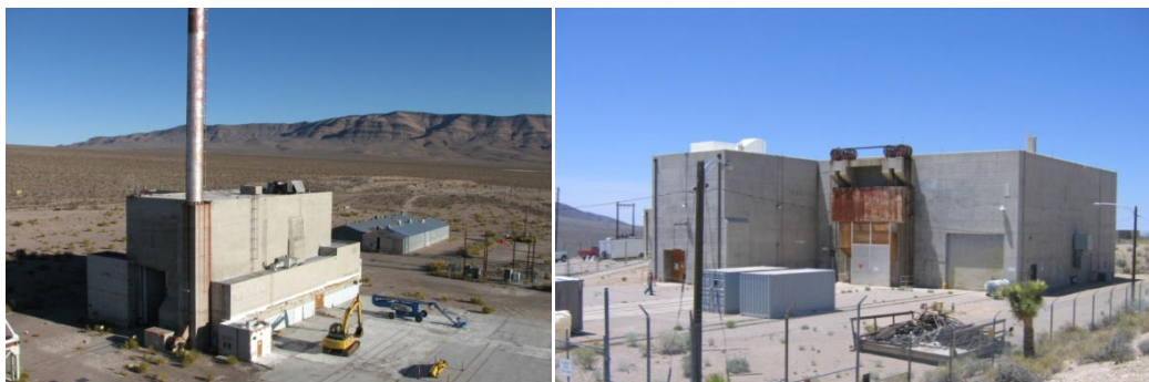
Figure 19. R-MAD Facility (left) and Pluto Facility (right)
