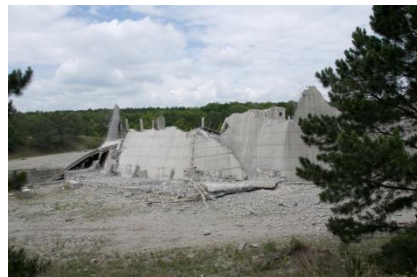
Cooling Tower (after)
