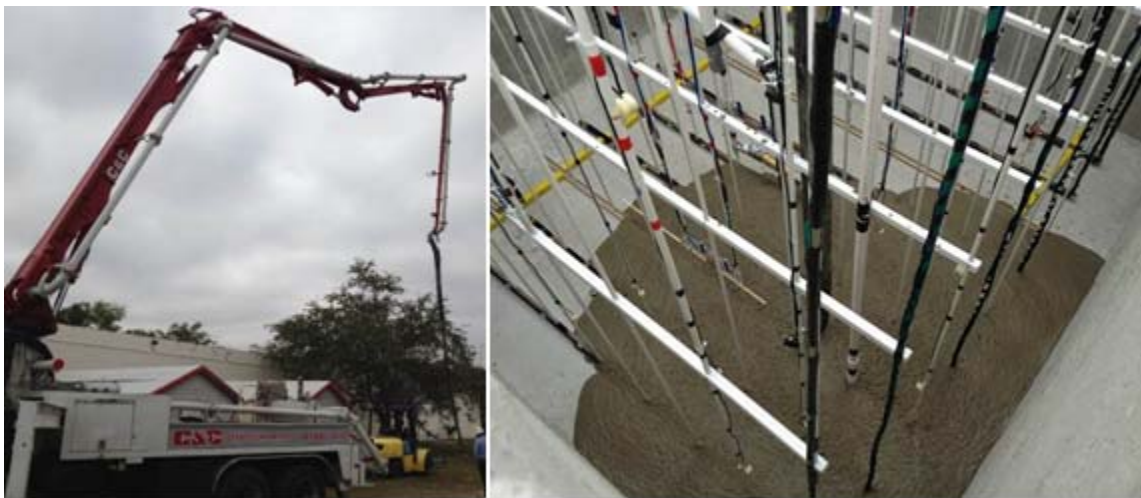
Figure 39. Grout pump and filling the cube with grout.
