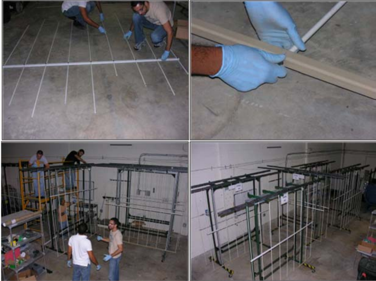
Figure 36. Assembly of ISDSN sensor racks and sensor racks support assemblies.
