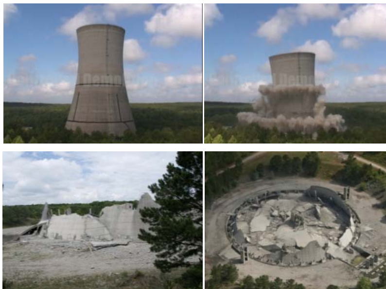
Figure 45. Implosion demolition of cooling tower at SRS.
