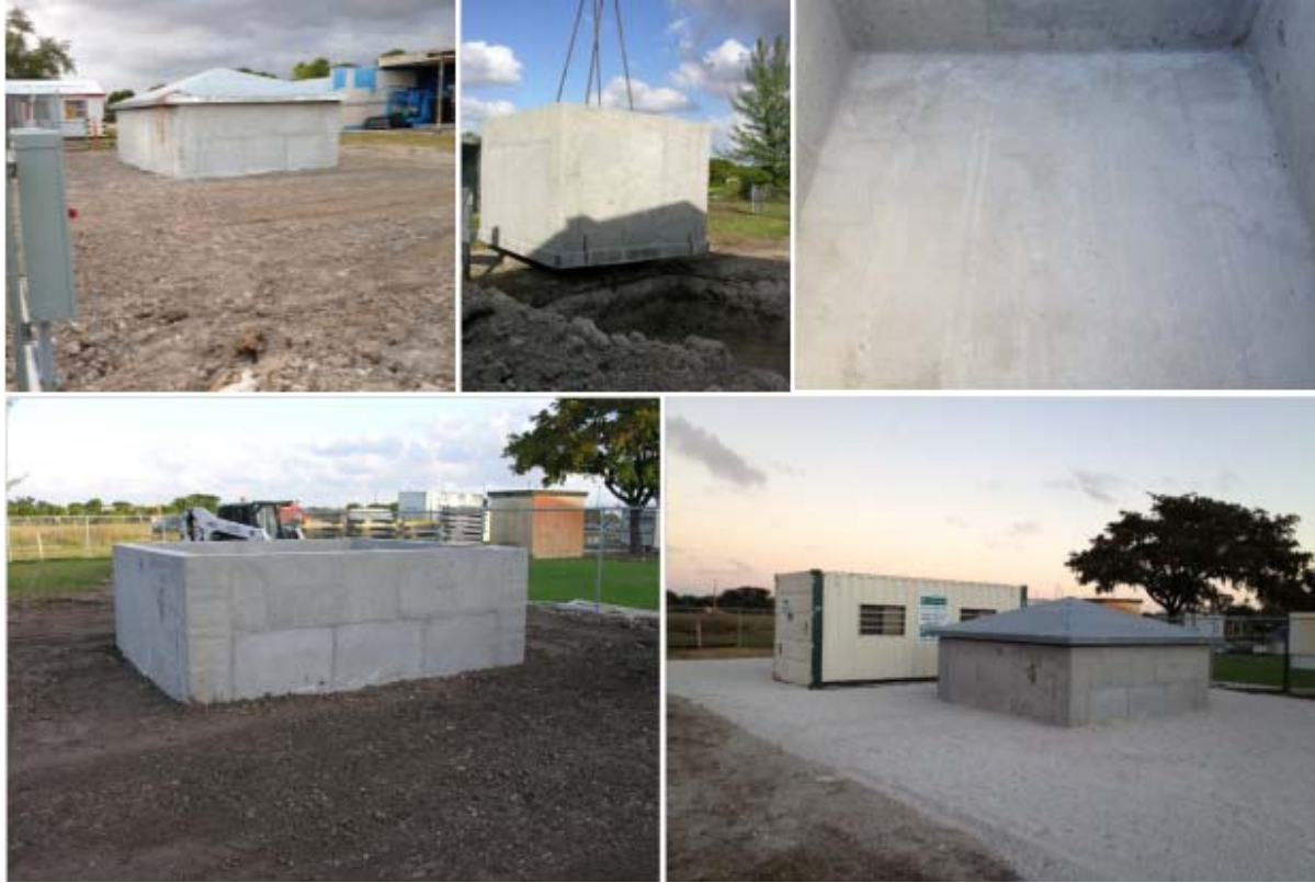
Figure 37. Preparation of the “cube” test site.
