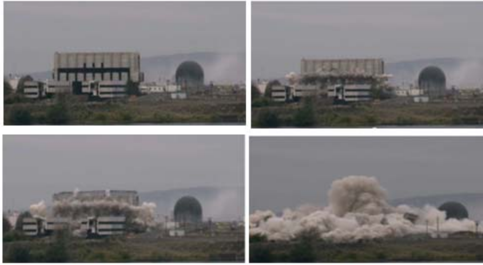
Figure 43. Demolition of Buildings 337 and 337B at the Hanford Site.
