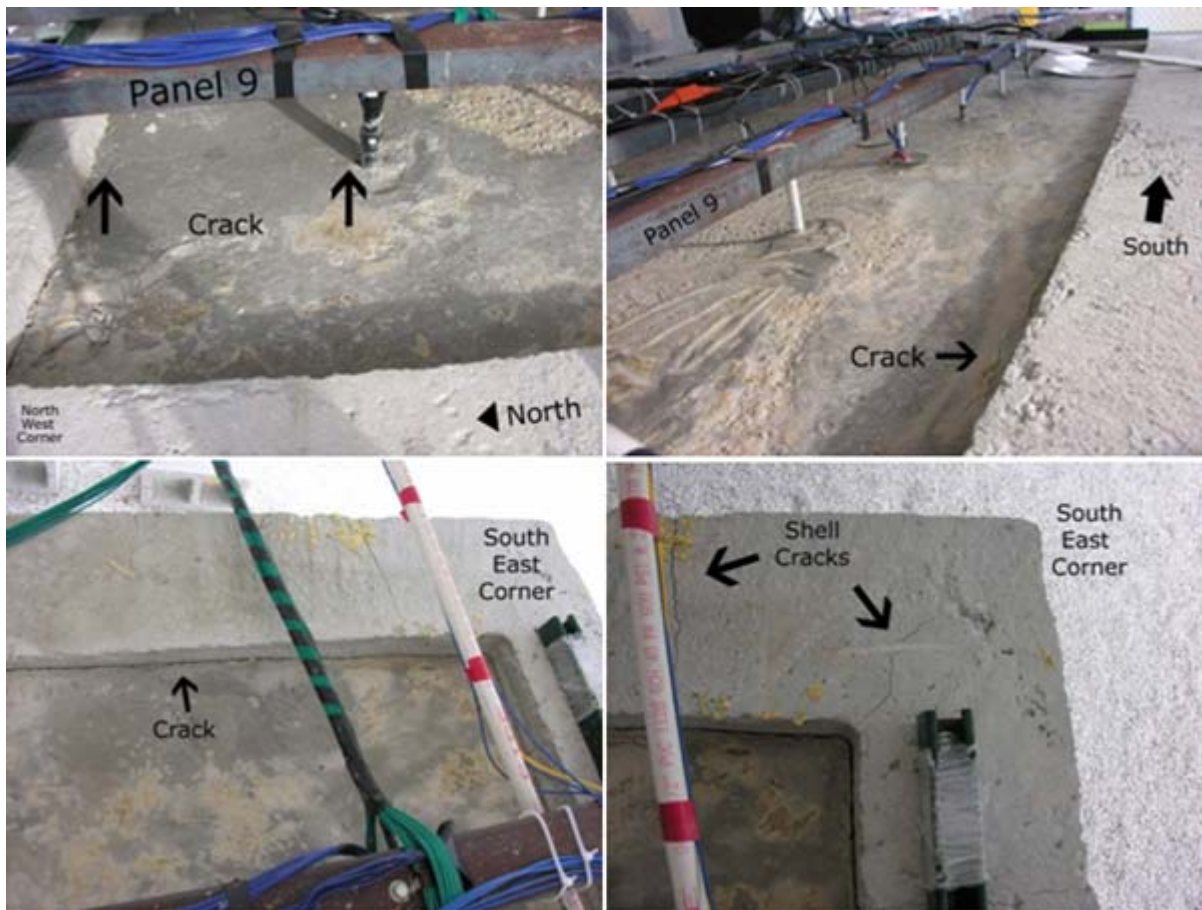
Figure 40. Cracks developing on cube surface.
