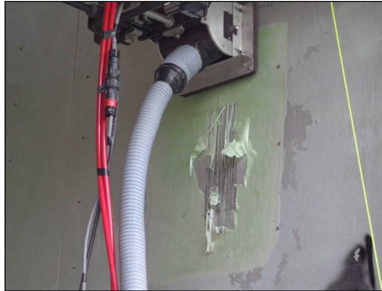
Figure 7. ICM remote platform using a brush with a vacuum shroud to remove strippable coating from vertical surface.
