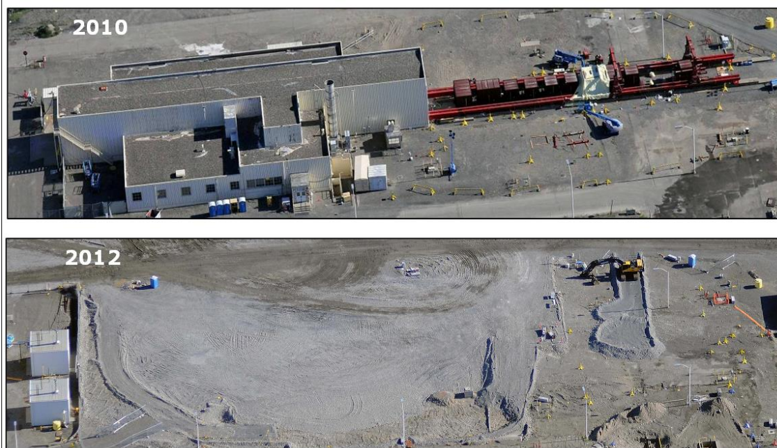
Figure 17. The Hanford Site 327 Building during hot cell removal activities and in 2012.
