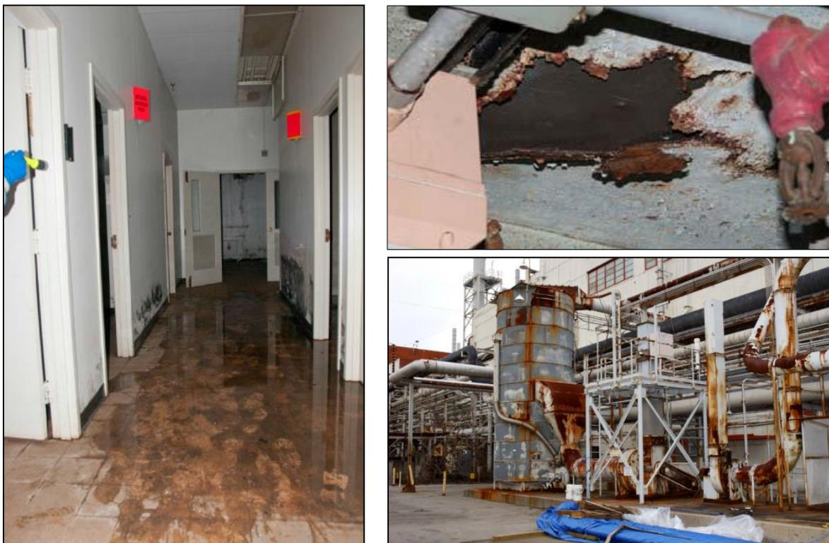
**Figure 35. Mold due to leaks (left), ceiling deterioration in Bldg 9206 (top right), and deteriorating infrastructure at Beta 4 (bottom right) (Source: Couchman-Griswold and Underwood 2014).**
