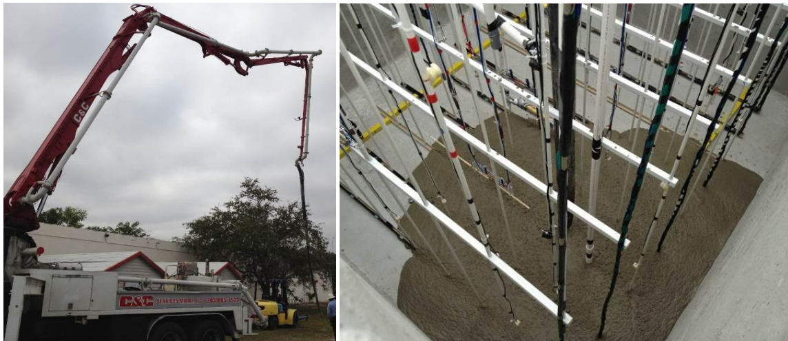
Figure 4-5. Grout pump and filling the cube with grout.
