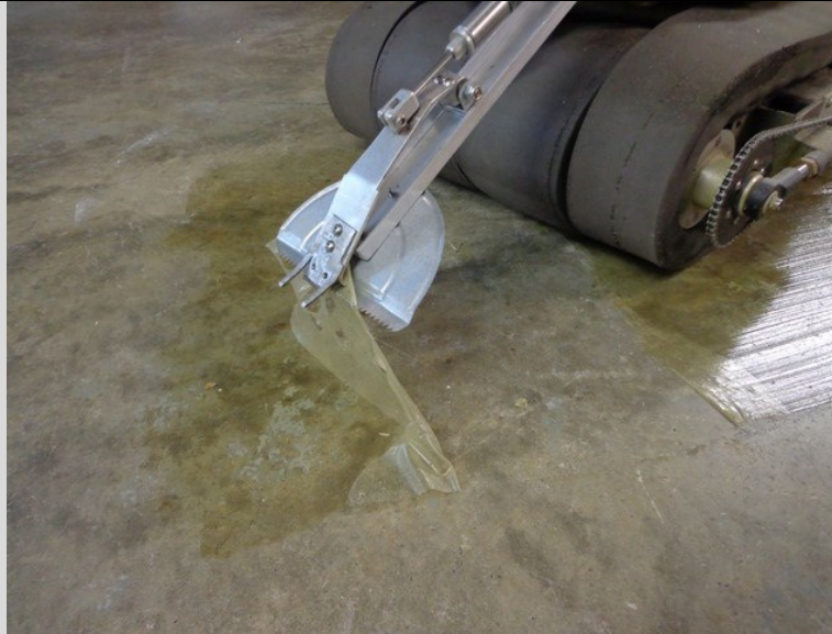
Figure 4-5 ICM remote platform with a gripper/scrapper tool to remove strippable coatings
