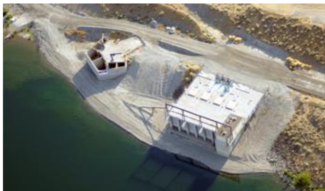
Figure 3-2. Earthen benches used to isolate structures from the Columbia River.
