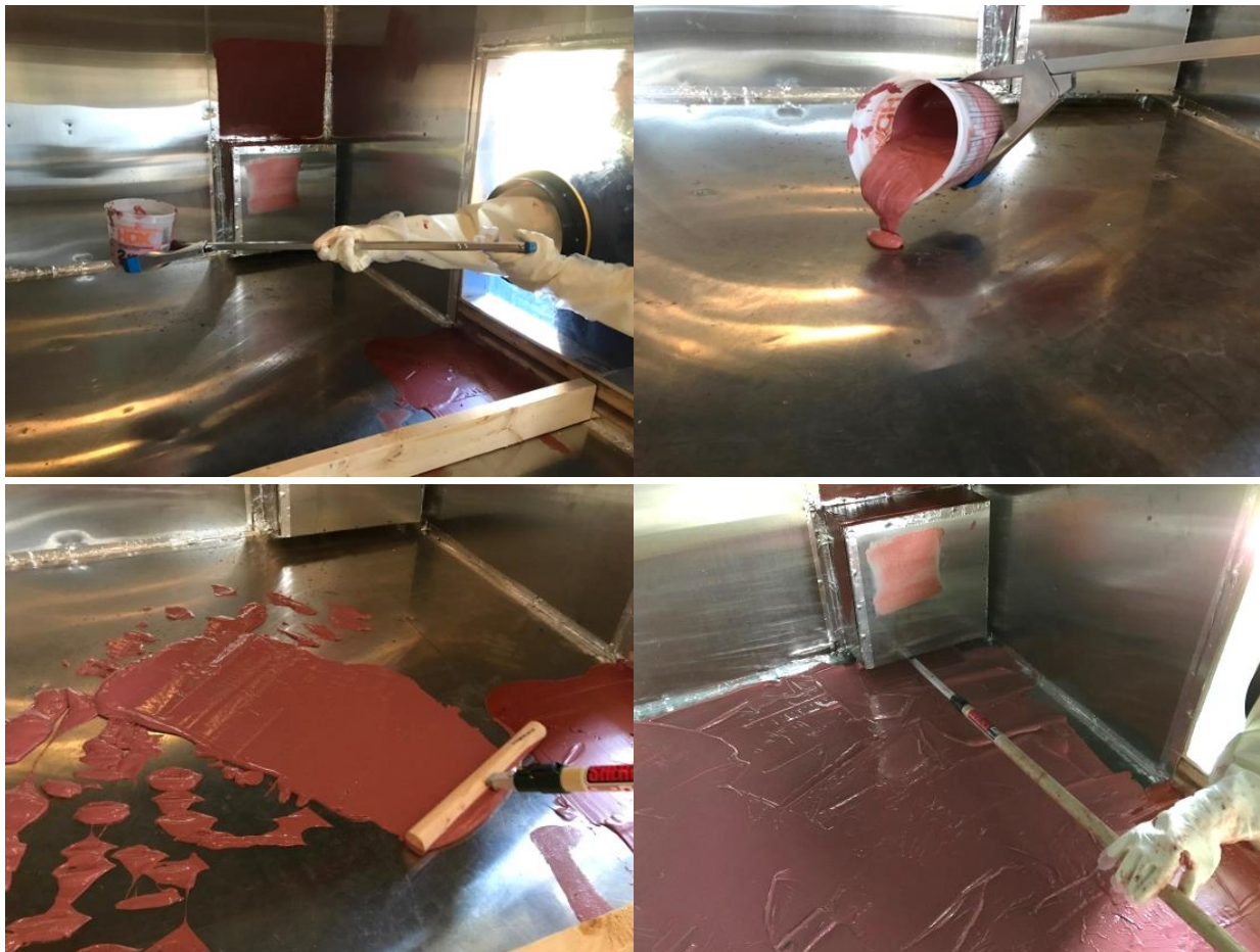
Figure 3-8. Slow pour method to apply IC to hot cell floor.
