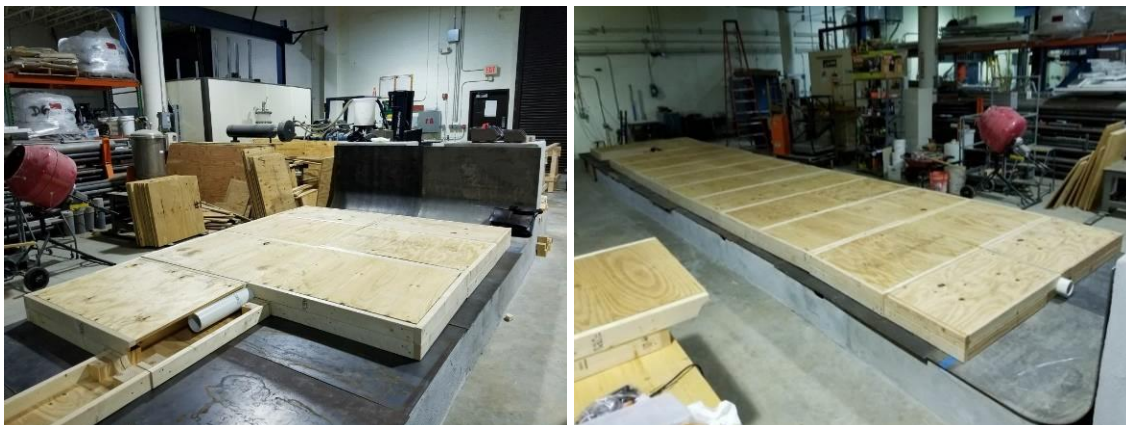
Figure 1-21. Plywood boxes that form the refractory.
