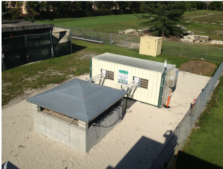
Aerial View of In-Situ Decommissioning Test Site at FIU
