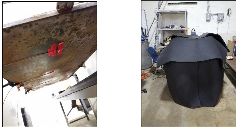
Figure 1-35. HSTs fixed under the plate (left) and tank covered with insulation (right).
