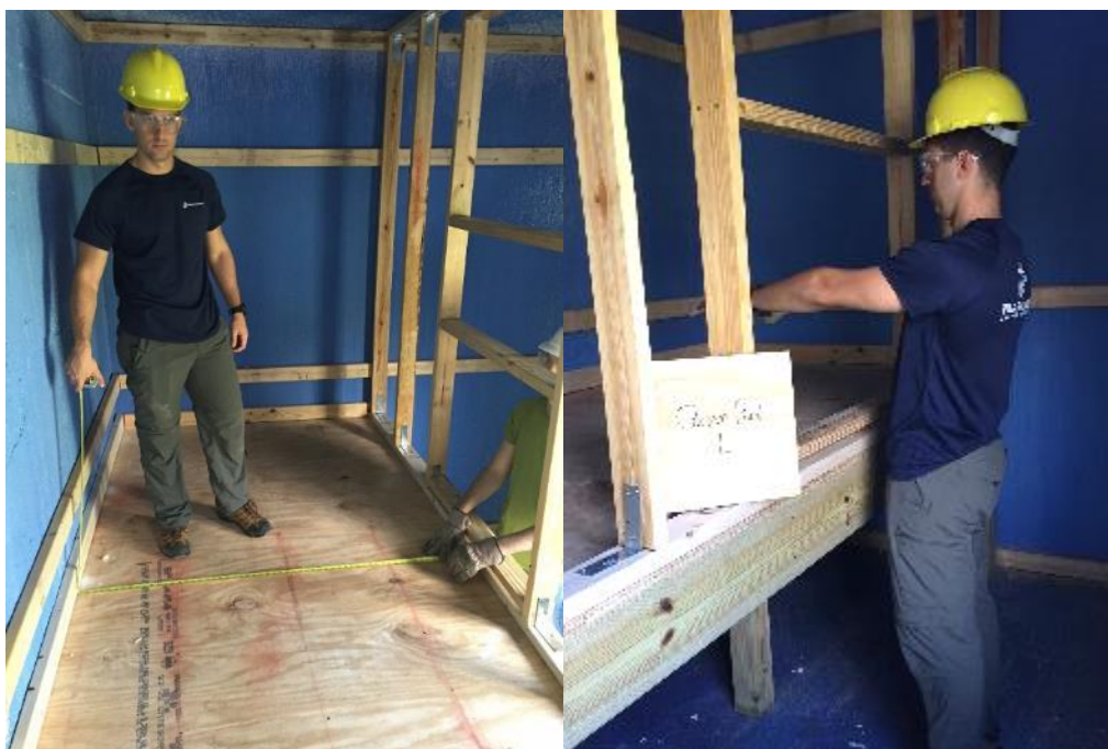
Figure 3-8. Hot cell width of 5 ft (left) and middle cell lower glove port (right).
