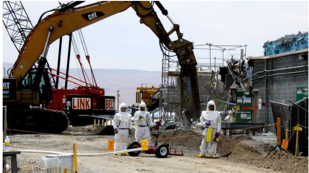
Demolition of the Plutonium Finishing Plant at the Hanford Site was halted in mid-December after radioactive dust was discovered far from the plant site. Vartabedian, R. (2018, April 16)
