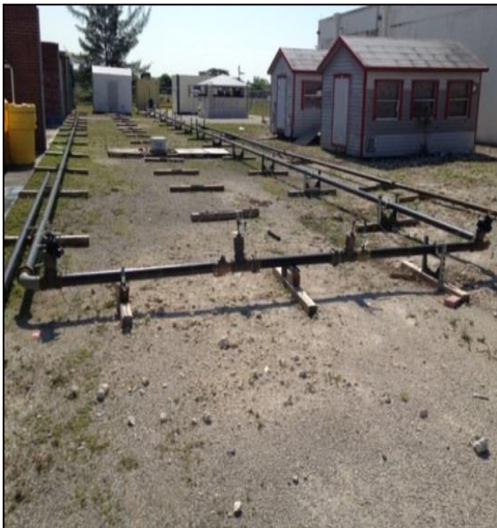
Existing 270-foot pipeline at FIU
