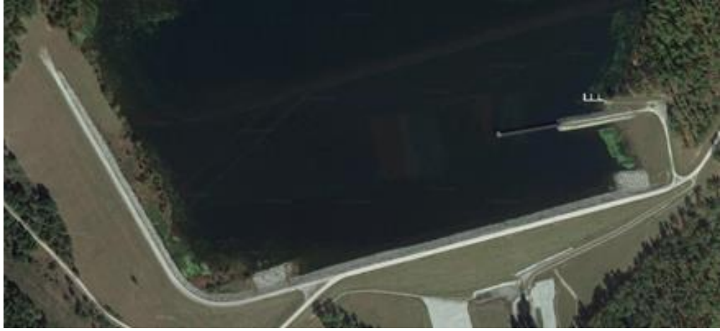
Steel Creek Dam
