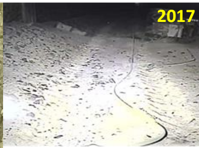
Accumulation of concrete products (e.g. \text{CaCO}_3 )
