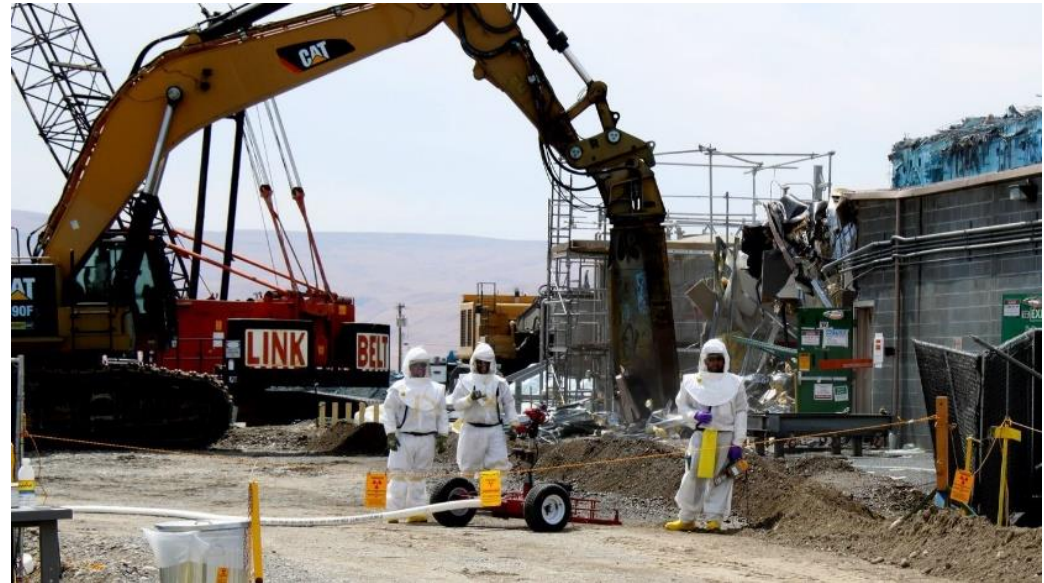
Demolition of the Plutonium Finishing Plant at the Hanford Site was halted in mid-December after radioactive dust was discovered far from the plant site. Vartabedian, R. (2018, April 16)
