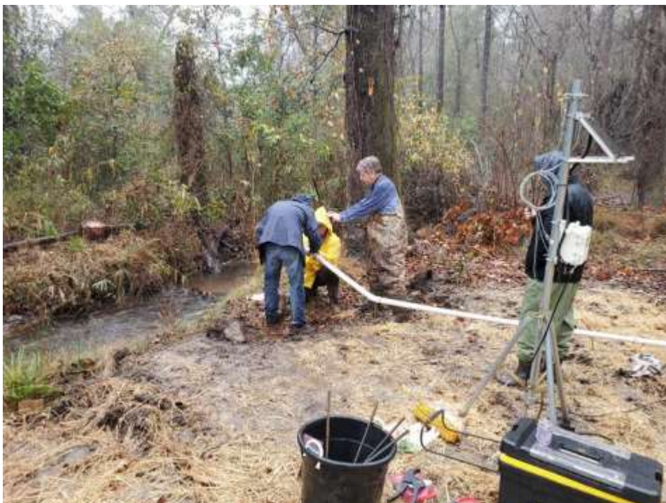
Figure 56. FIU and SRNL collaborators positioning the sensor/probe at the end of the PVC piping prior to placement in the stream.
