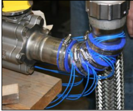
Figure 121. Installed Pipe Wrap™ system on a 2” diameter pipe [1].
