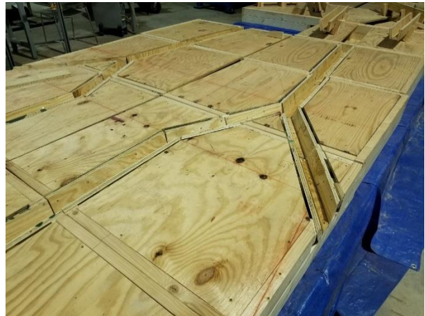
Figure 77. Framing for the refractory slots.
