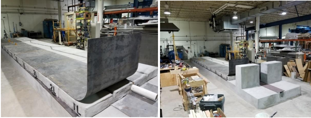
Figure 80. Construction of the full-scale HLW DST test bed.
