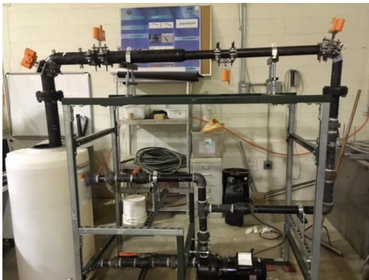
Figure 81. Erosion Pipe loop with sensors.
