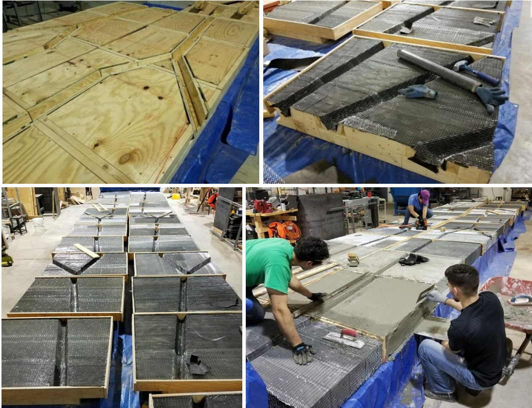
Figure 79. Refractory channel construction.
