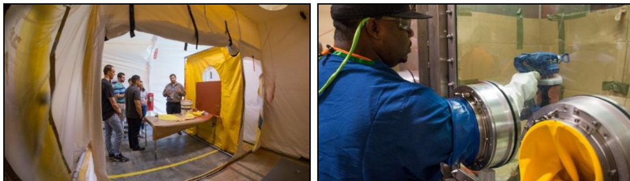
Figure 16. IC application demonstration at the SRS 235-F Process Cell Mock-up & Training Facility.
