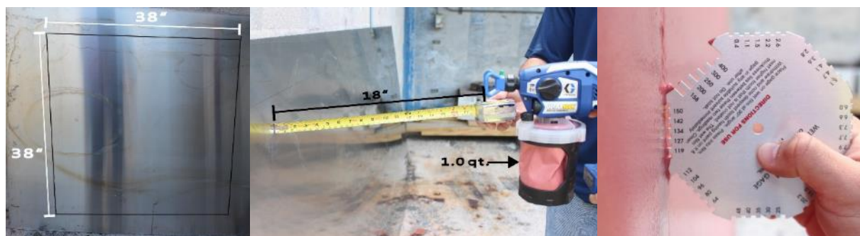
Figure 11. Confirmation testing of coating thickness with multiple applications of IC.
