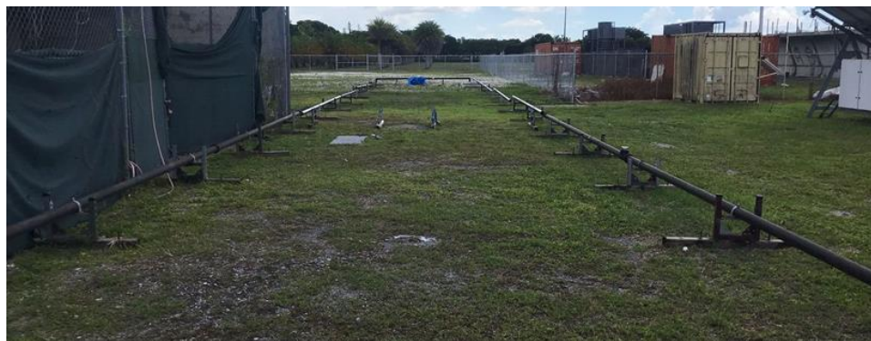
Figure 4. Constructed 330-foot extension used for flushing.
