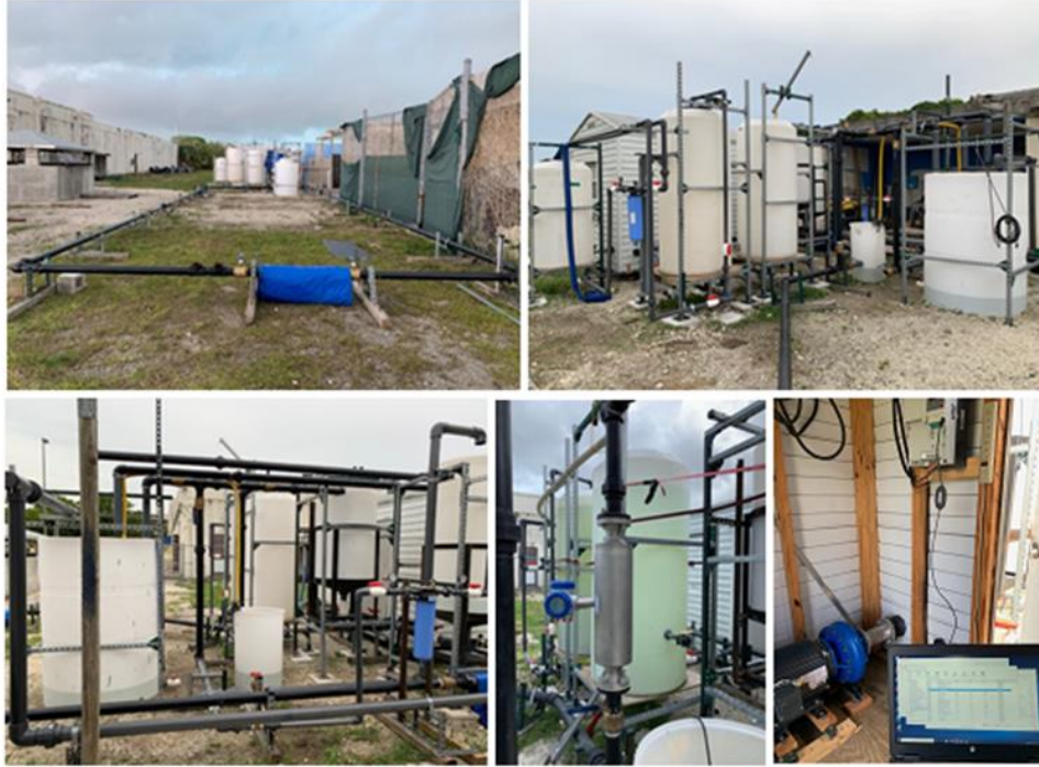
Figure 2. Constructed 165-foot pipeline for flushing experiments.
