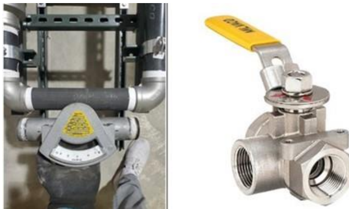
Figure 98. Flow meter to replace 12-inch pipe section (left) and 3-way ball valve (right).
