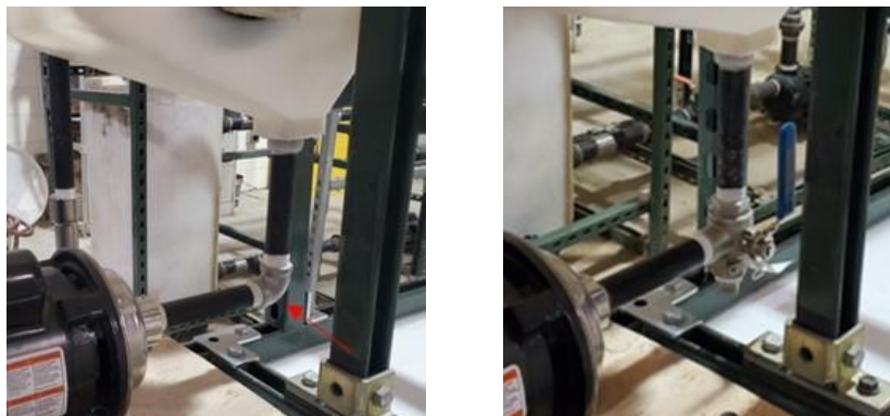
Figure 99. 3-Way ball valve location (red arrow) (left) and installation (right).
