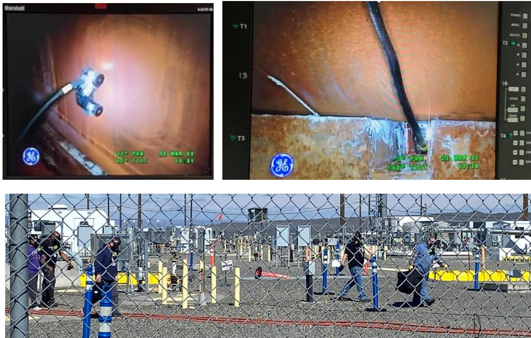
Figure 14. Hanford AP-105 DST deployment.
