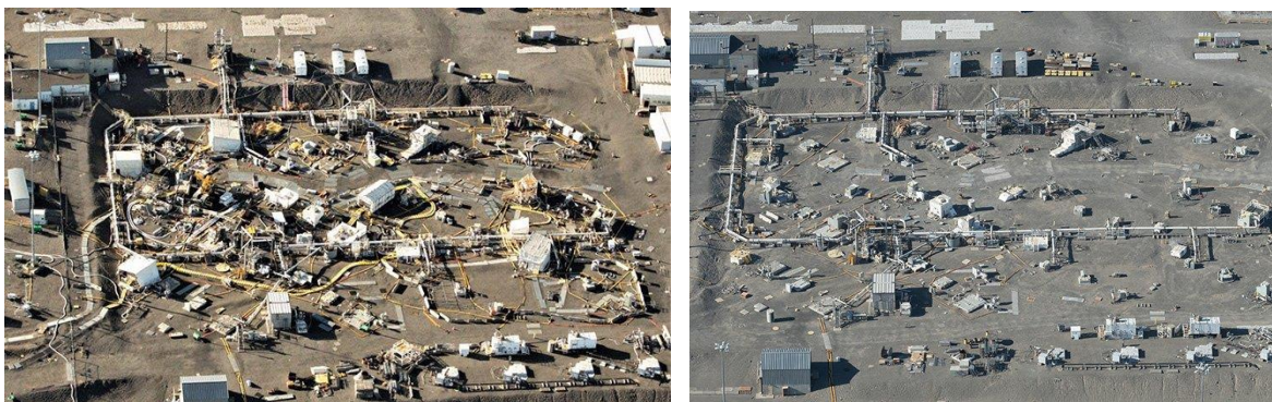
Figure 70. Hanford's Tank Farm retrieval operations in September 2016 (left) and 2018 (right).
