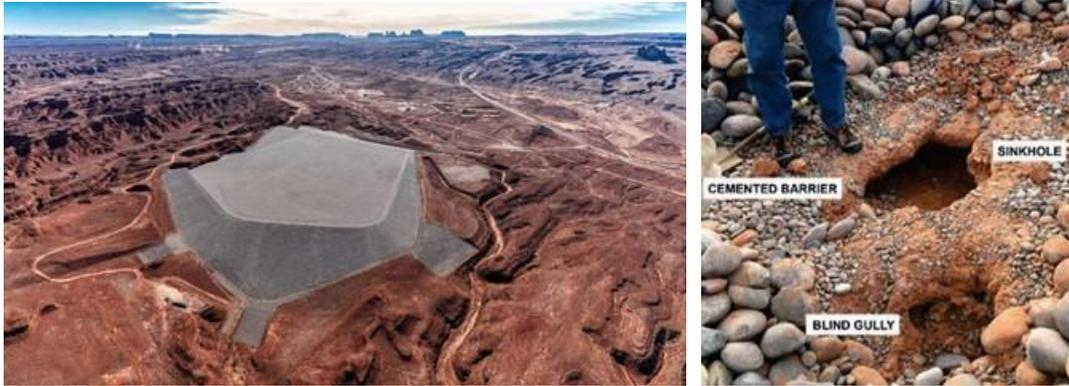
**Figure 36. Erosion issues at the Mexican Hat Disposal Cell in Utah.**
