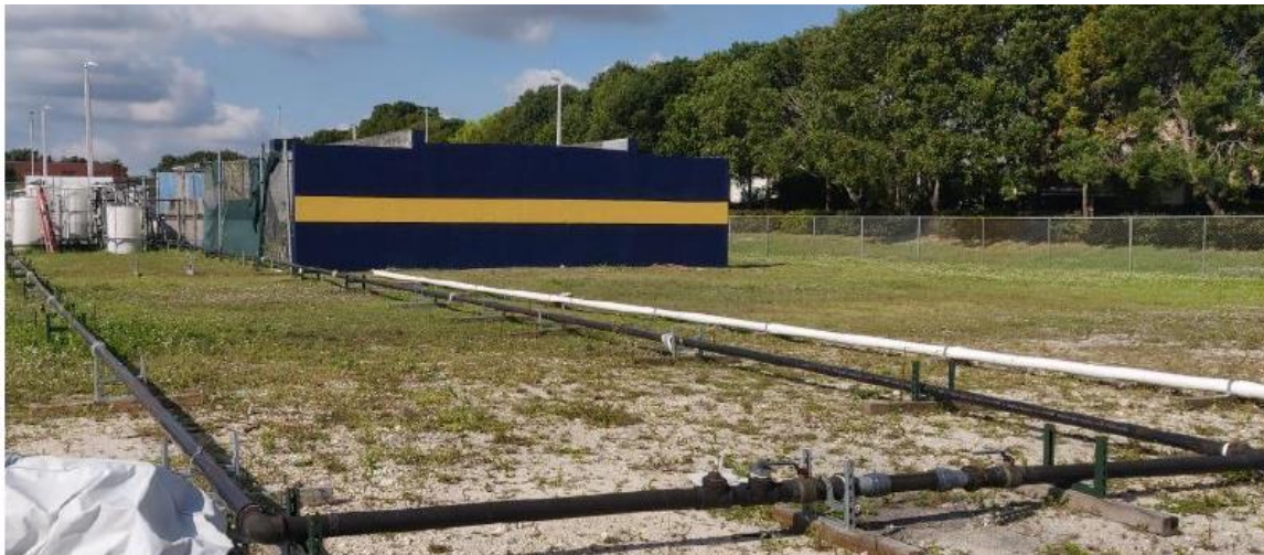
Figure 3. Constructed 330-foot extension used for flushing.
