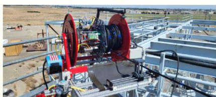
The "Lateral Gamma Scanner" crawler bot is lowered down the pipe and retracted using a reel and cable system.
