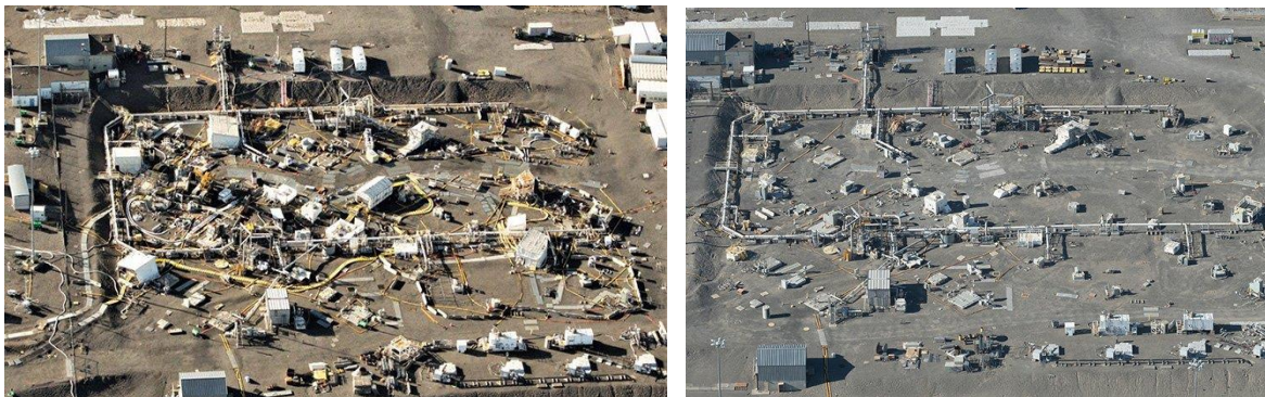
Figure 19. Hanford's Tank Farm retrieval operations in September 2016 (left) and 2018 (right).
