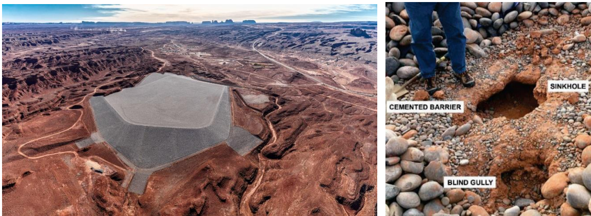
Figure 18. Utah Mexican Hat Disposal Cell (left) and subsurface erosion discovered in 2017 (right).
