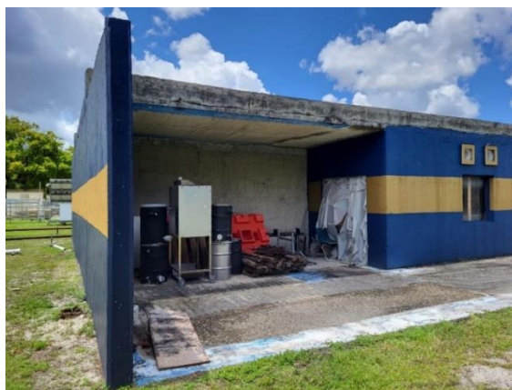
Figure 18. Outside testing facility and area of mockup construction.
