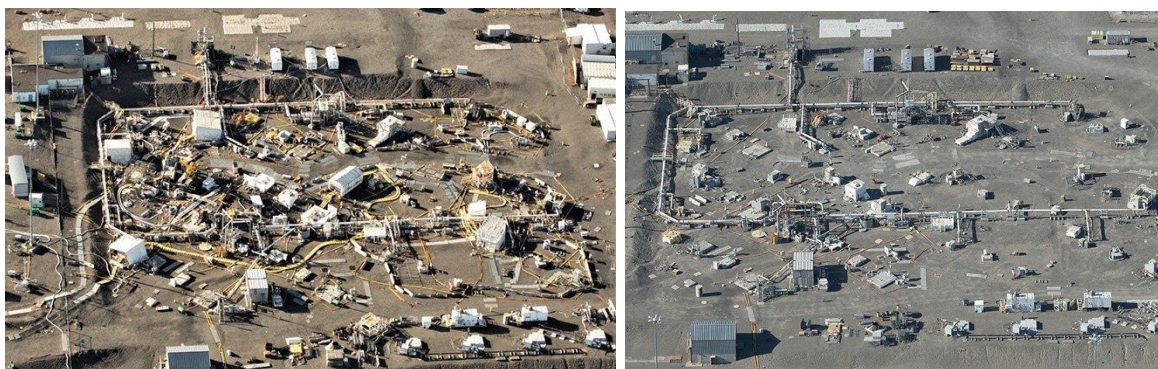
Figure 21. Hanford's Tank Farm retrieval operations in September 2016 (left) and 2018 (right).
