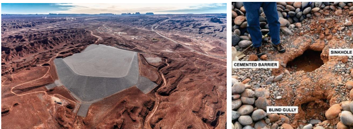
Figure 6. Utah Mexican Hat Disposal Cell (left) and subsurface erosion discovered in 2017 (right).
