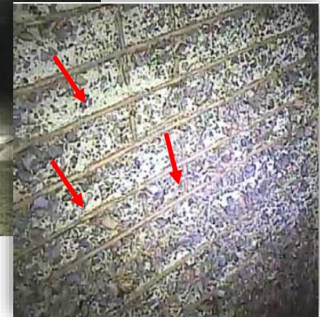
Degraded concrete exposing the steel rebar (red arrows).
